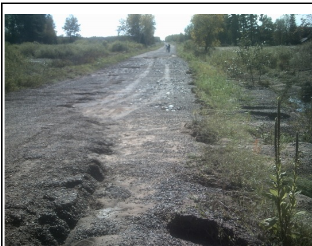
Figure 3.2 Road Washout September 2010
