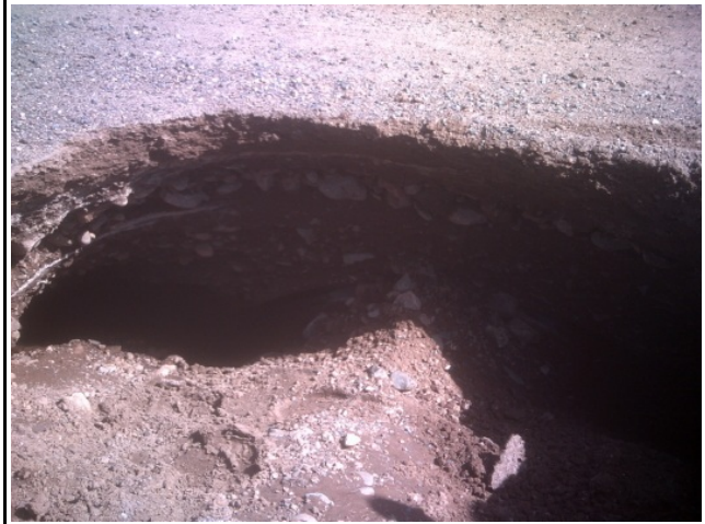
Figure 3-3 Washout under pavement September 2010
